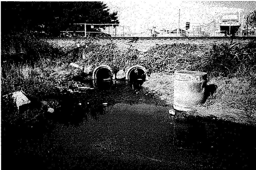
W-1 View downstream, twin culverts under BNRR tracks directing Edmonds Marsh drainage to Puget Sound (10/20/98).
