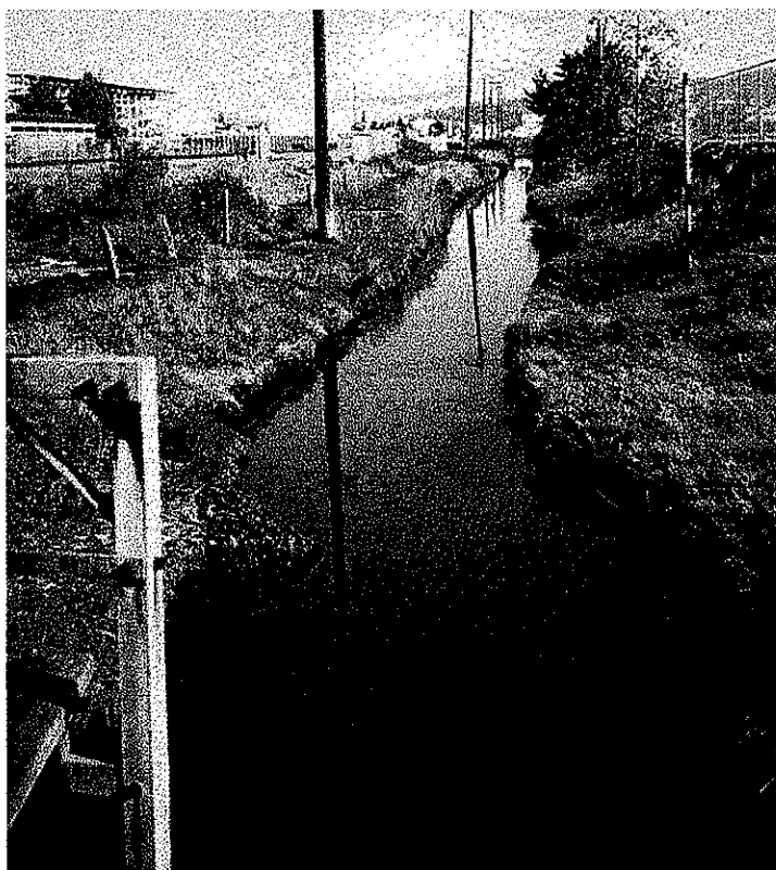
W-2 Channelized lower portion of creek along Admiral Way (10/20/98).
