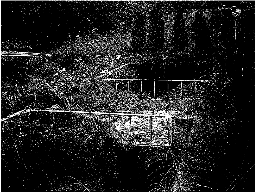
P-3 Perrinville Creek stormwater overflow.
