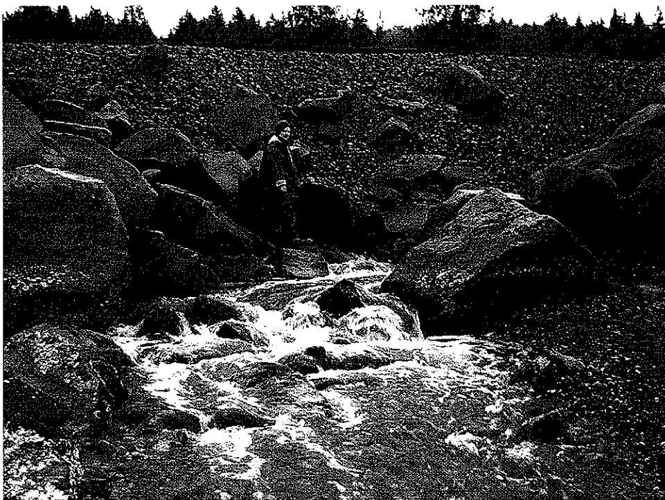
P-1 Perrinville Creek, downstream of culvert under BNRR tracks.
