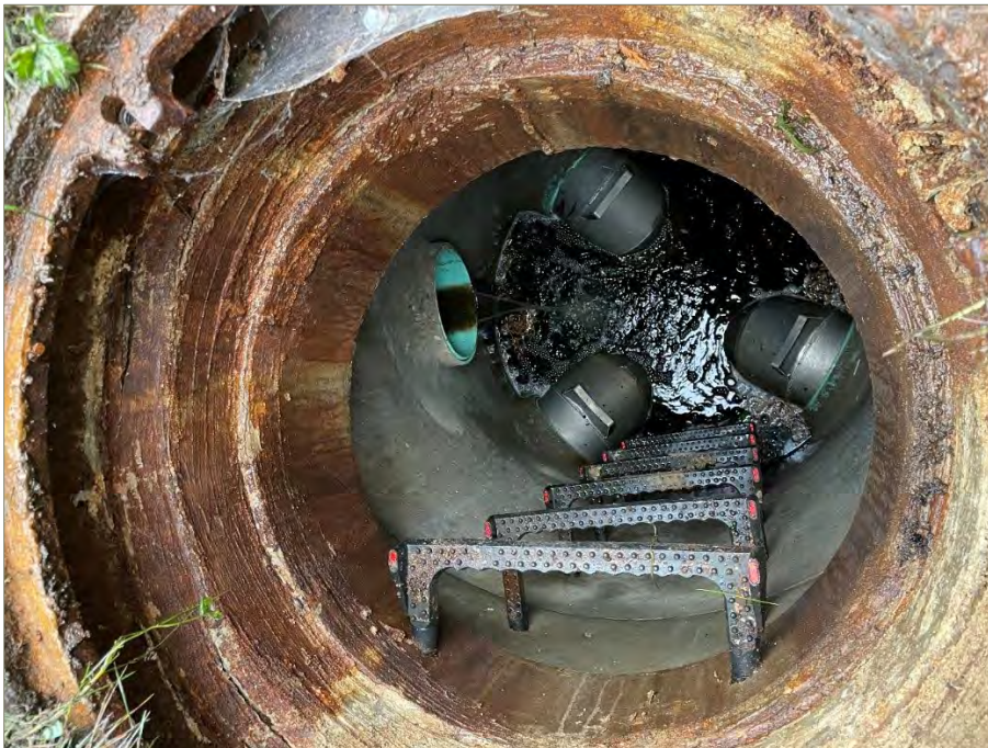
Exhibit 1: View of the interior of SDCB 105. The stormwater sample was collected as water exited the green pipe without the elbow. The pipes with downturned elbows distribute water to Wellfield 1 dry wells.
