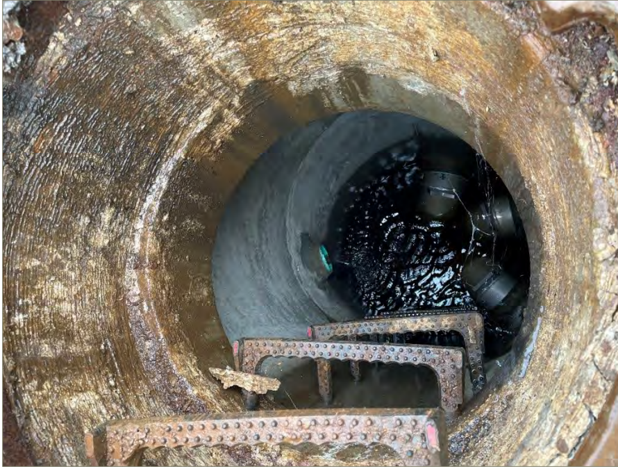
Exhibit 1: View of the interior of SDCB 105. The stormwater sample was collected as water exited the green pipe without the elbow. The pipes with downturned elbows distribute water to Wellfield 1 dry wells.
